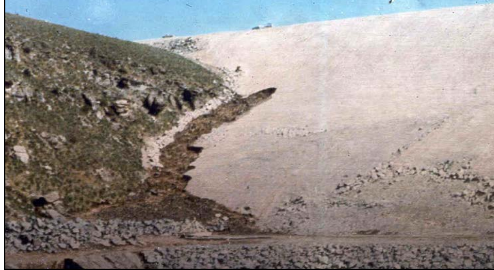
Teton Dam 1976, 11 Fatalities - Initial Filling Internal Erosion
