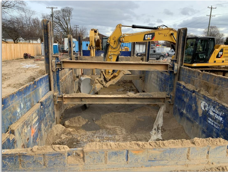
Removal of 10,800 tons of contaminated soil (2,200 tons classified as Hazardous Waste)
