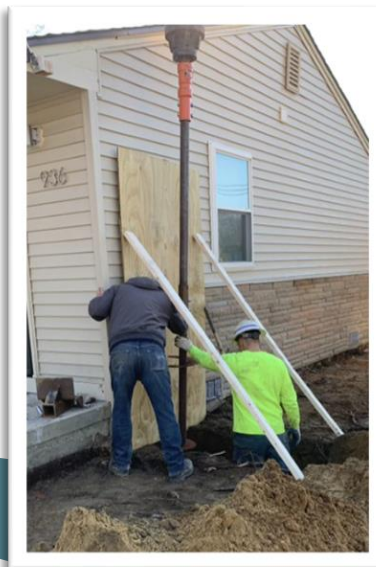
Installing vapor mitigation systems
