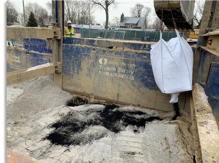
Mixing absorbent material into backfill to treat groundwater
