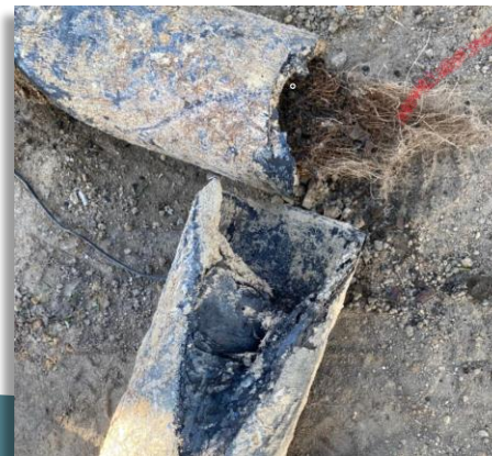
Damaged sewer pipe
